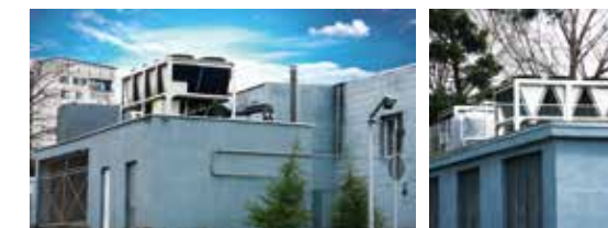
Police Station Vazisubani
