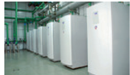
Seven Thermia Robust Eco units connected together.
