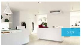
**Ceiling suspended unit FXHQ-A:** For wide rooms with no false ceiling nor free floor space
